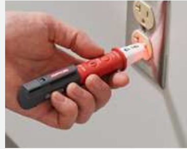
Test wall sockets for AC voltage
