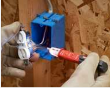
Test wires for AC voltage
